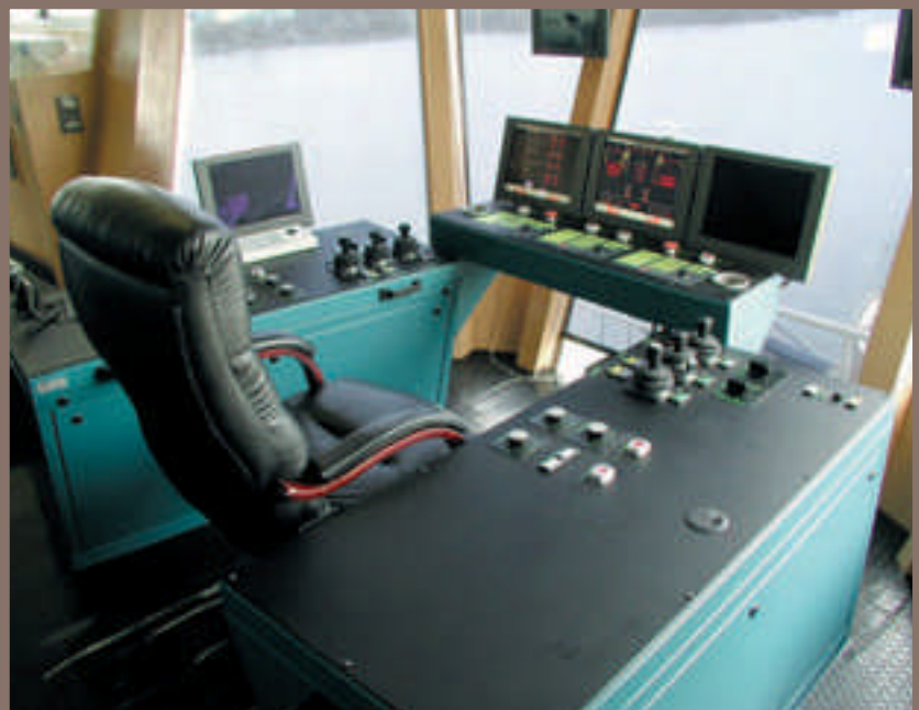
Dredge operators' new controls
